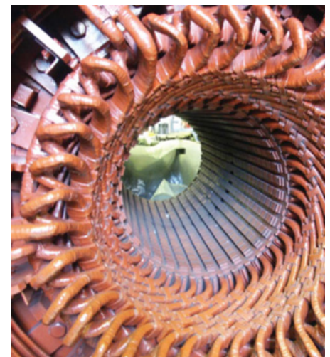
5-megawatt steam turbine
