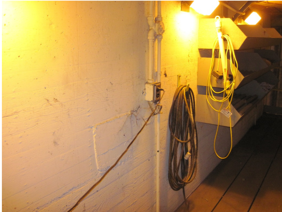
Lower Monumental Headgate Repair Pit: lighting and extension cords.
