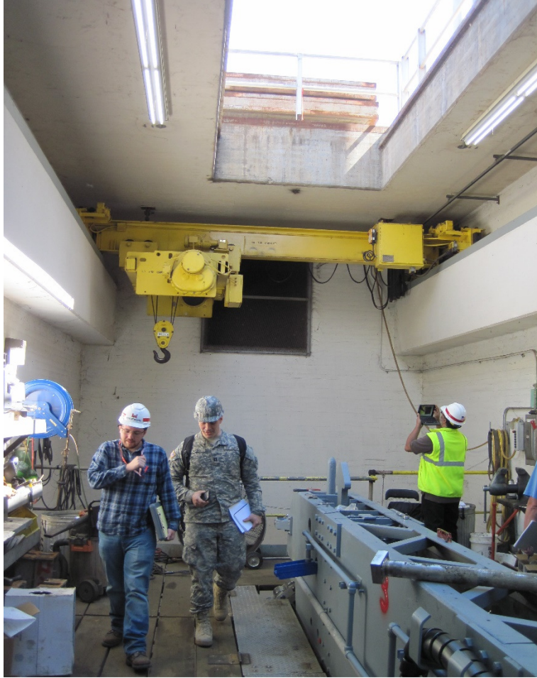
Lower Monumental Headgate Repair Pit, including wooden planks.
