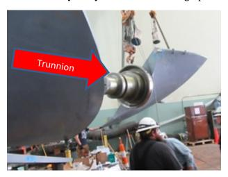
Photo 1-Removal of Turbine Blade
