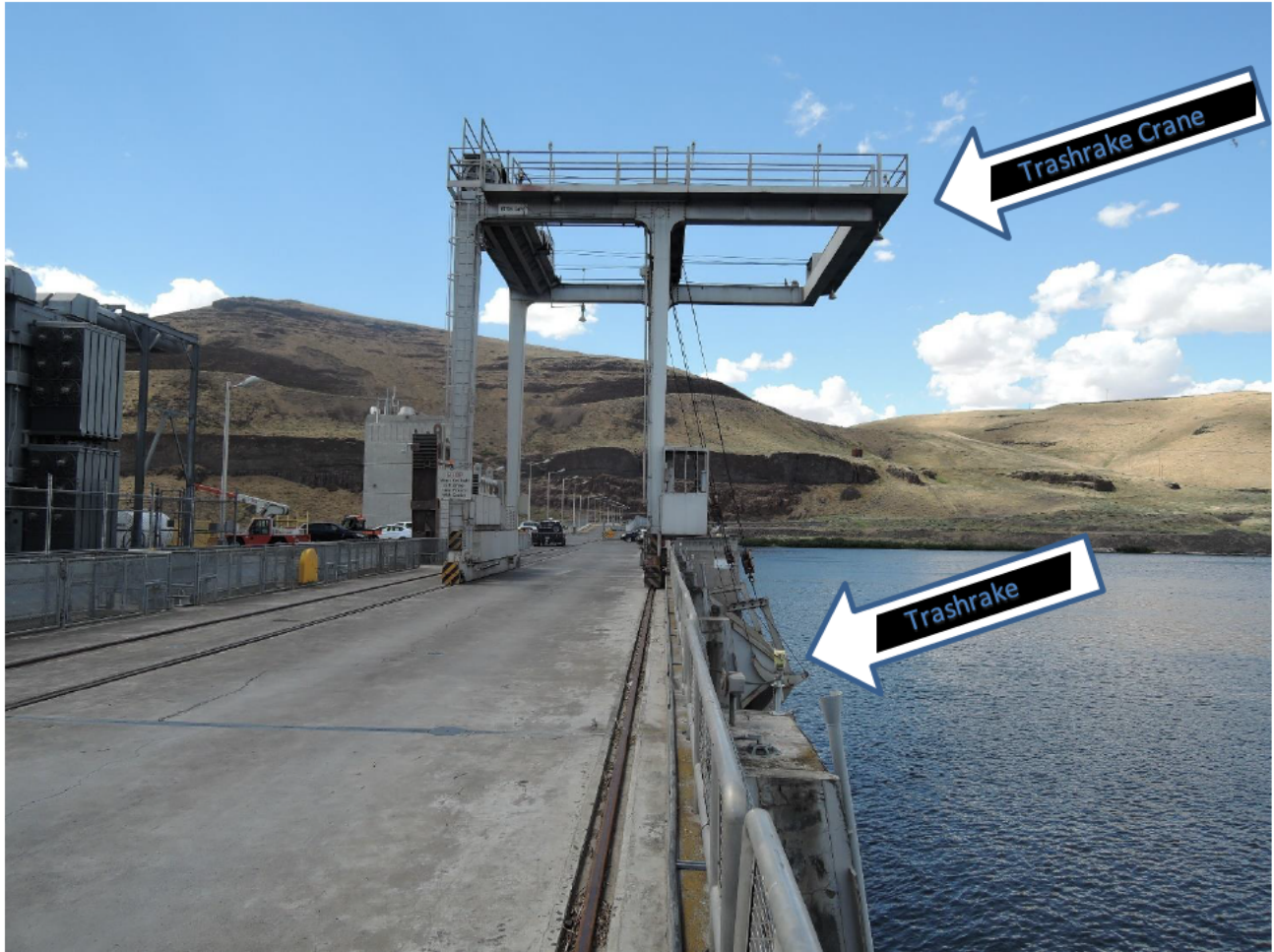
Little Goose dam and reservoir project's Trashrake Crane and Trashrake
