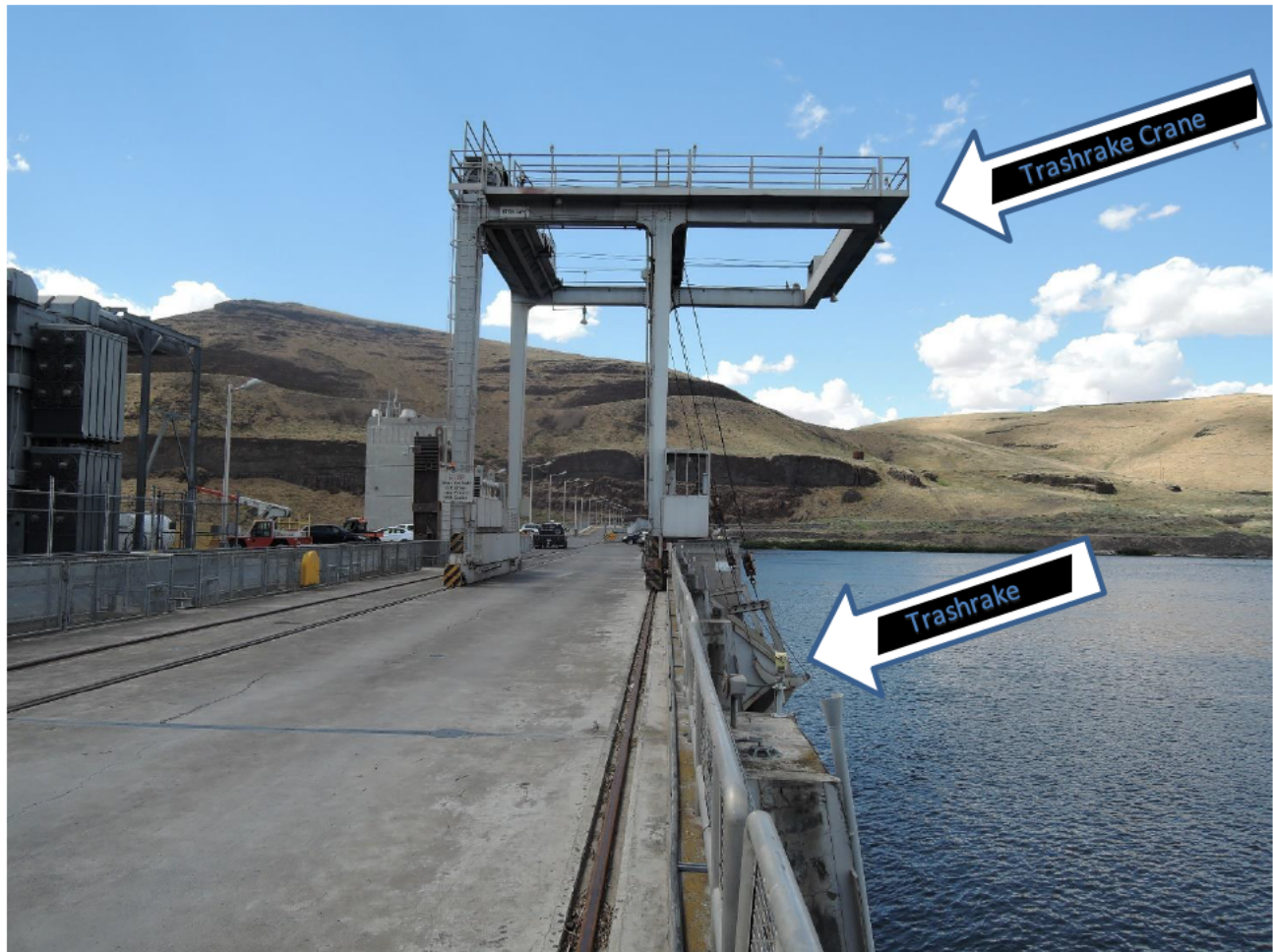
Example of a Trashrake Crane and Trashrake (Little Goose dam and reservoir project)
