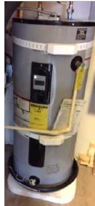
Figure 19. Tank Installed at Site 10
