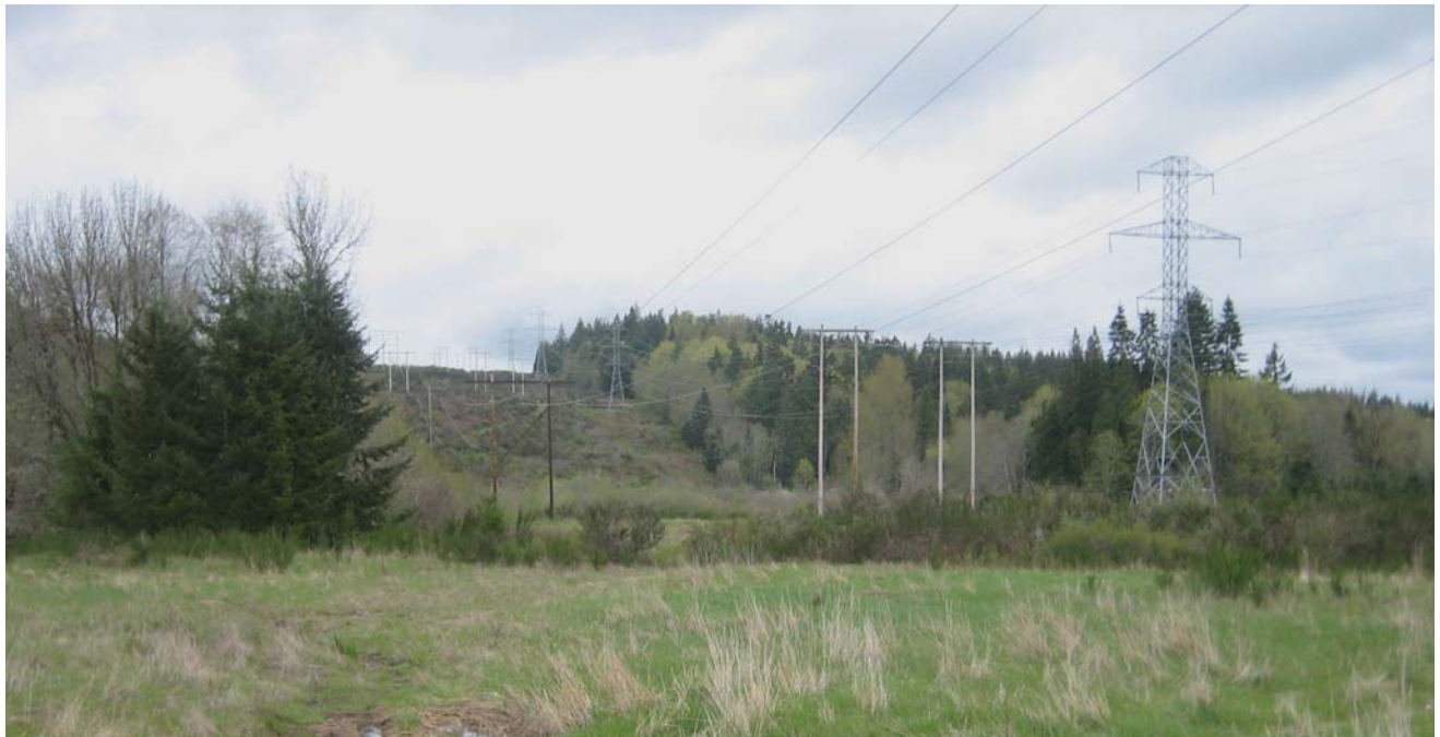
Figure 7 Existing Olympia-Shelton No. 1 115-kV Line near Center of the Corridor (looking north)
